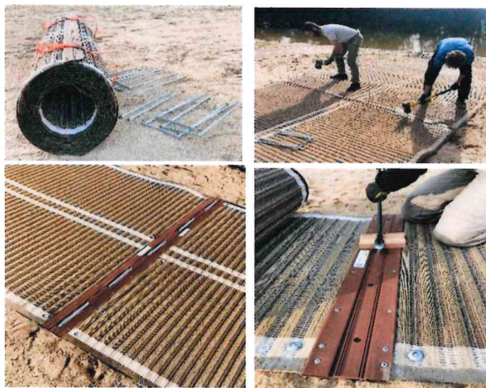
All anchors are provided with the mat. Depending on the dimensions of the mats, the number of eyelets and anchors varies.
